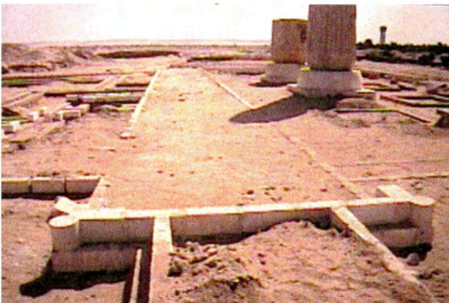
Small Aten Temple: the foreground stonework is reconstructed to desired height and the space between in being filled.
